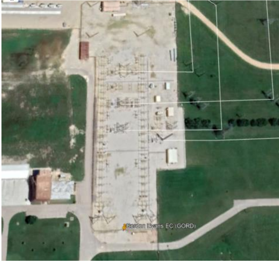
Figure 33 – Gordon Evans 138kV Substation
